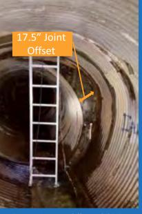
Figure 9: Joint Offset of CMP at Sinkhole Location
