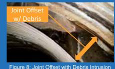
Figure 8: Joint Offset with Debris Intrusion
